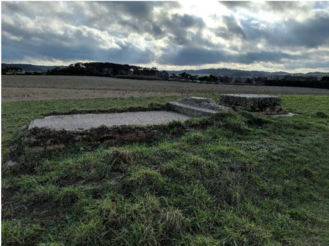
Plate 23.1.4-33 View of concrete building base, looking south.
